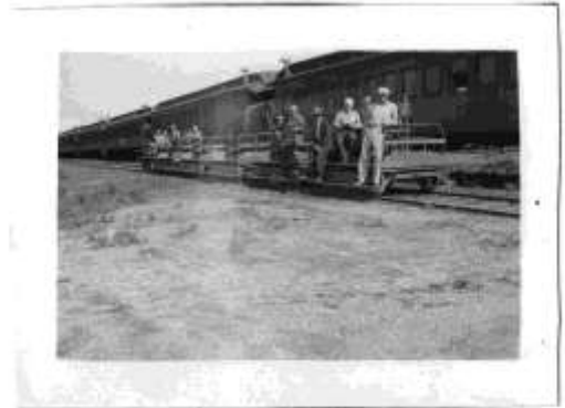
(5 work car trains behind crew posing on trailers)
